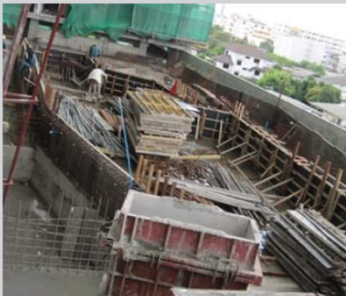
Concrete Structure from Wooden Framework 90-120 days
