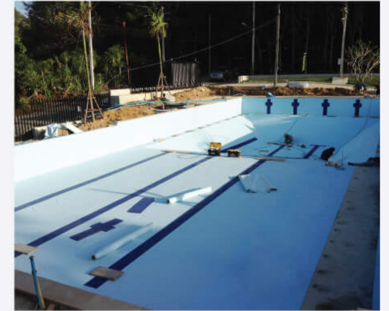
Liner Pool No leaking 100%
