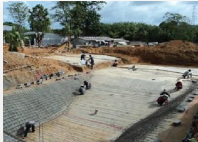
2. Reinforced Rebar Slab and Levelling Blocks
