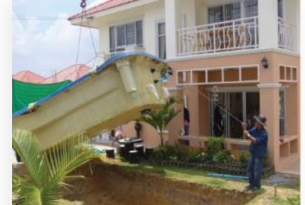
4. The Pool is lowered into the hole
