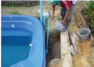
6. Begin filling with water and back filling
