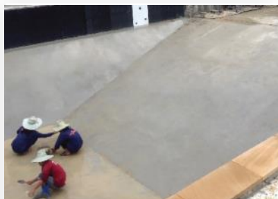
6. Laying coping stones and then ready for PVC lining
