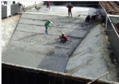
5. Pours concrete into pool slab and wall in a single process
