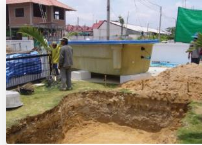
3. Hole Surface Preparation and Sand Bed
